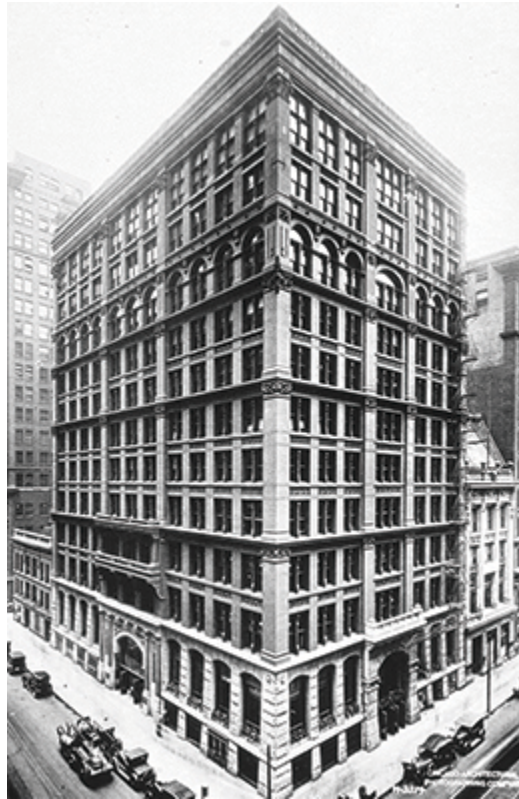
Figure 4.5 While the technology existed to engineer tall buildings, it was not until the invention of the electric elevator in 1889 that skyscrapers began to take over the urban landscape. Shown here is the Home Insurance Building in Chicago, considered the first modern skyscraper.
