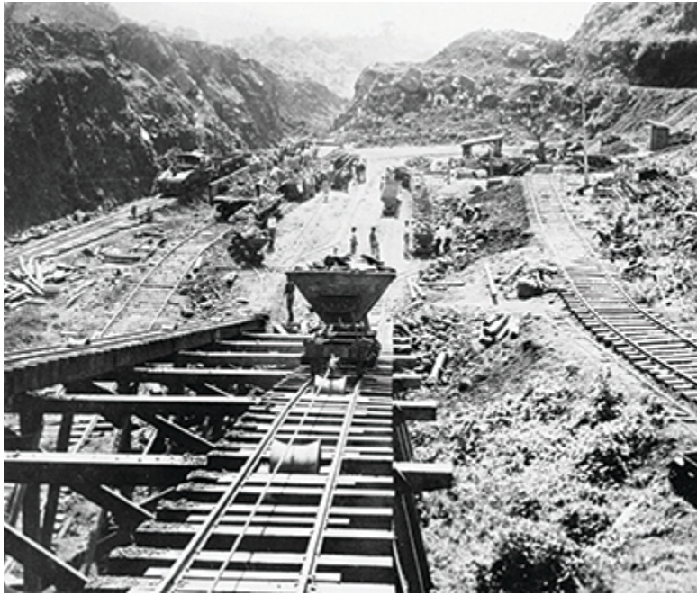
Figure 7.15 Recurring landslides made the excavation of the Culebra Cut one of the most technically challenging elements in the construction of the Panama Canal.
