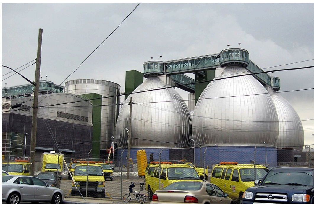
Figure 13.5 Egg-shaped “digesters” at the Newton Creek Wastewater Treatment Plant; Author | Jim Henderson; Source | Wikimedia Commons; License | Public Domain.
